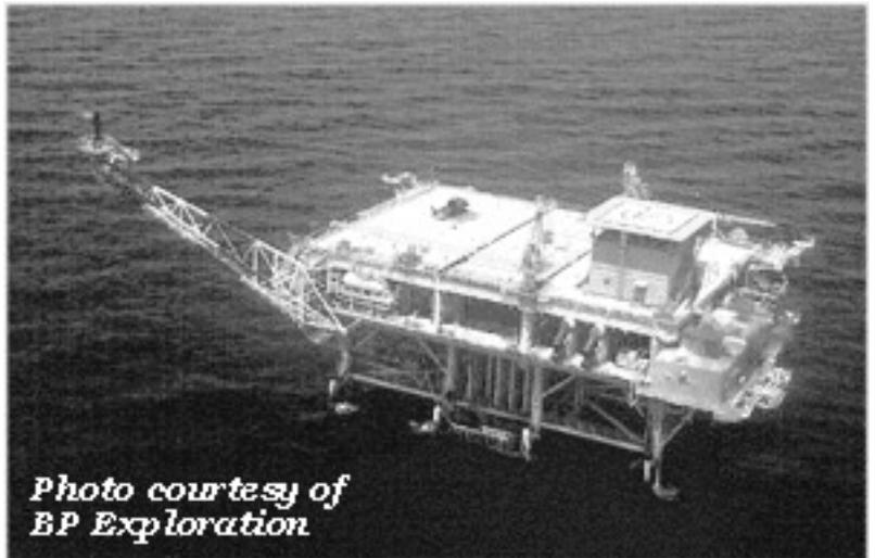
Offshore platforms are usually constructed from steel, but sometimes they can be built of concrete. When most of the oil has been recovered, the offshore platform is removed. Some are taken to shore to be dismantled and recycled. Others are converted into artificial reefs to enhance fishing.
