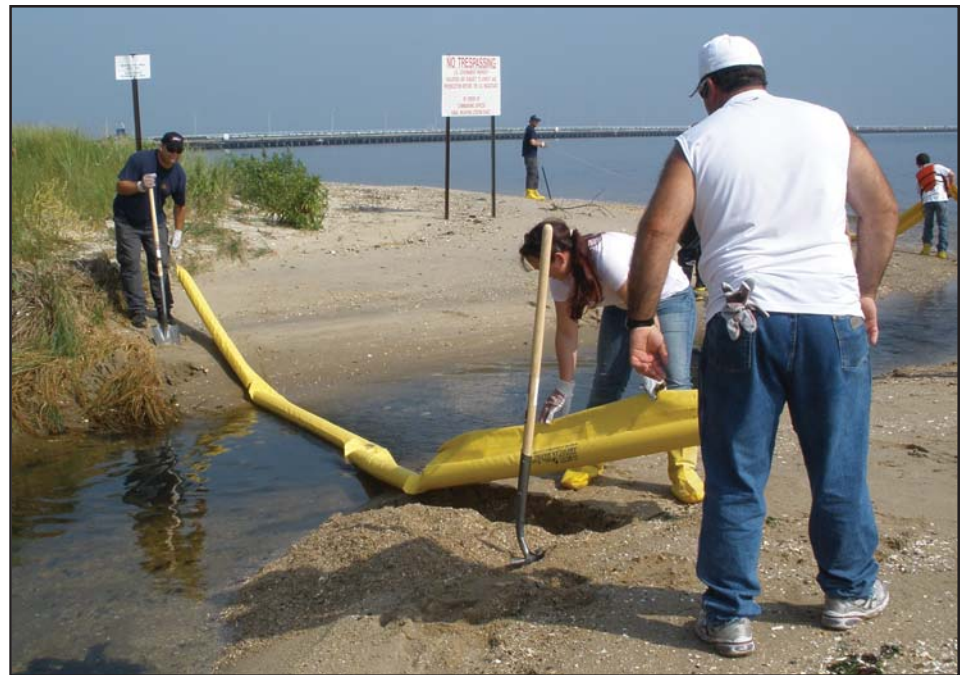
Emergency Response Technicians from the CHS Cooperative deploy boom at the mouth of the outfall to divert oil during the hands-on bay spill scenario.
