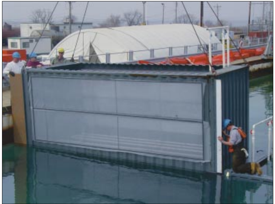
Dispersant filter chambers are lowered into the basin
