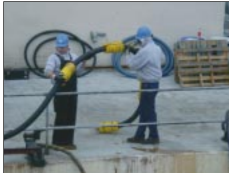
Uncoiling a skimmer discharge hose.
