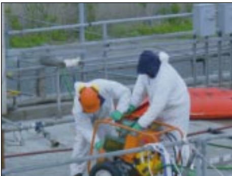
Assembling a hydraulic power pack
