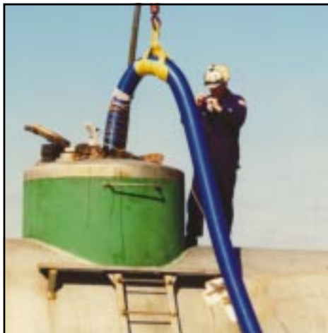
Oil being transferred to the rail car
