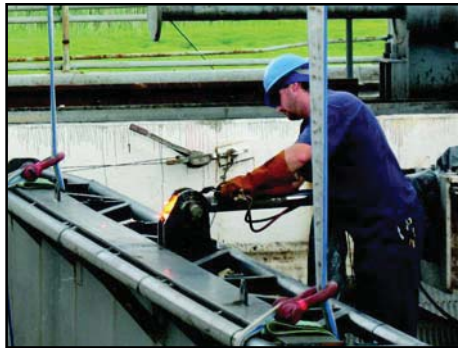
Technician Tom Schmidt prepares wave flaps for removal.
