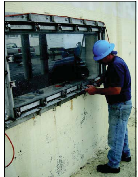
Test Director Dave DeVitis installs custom designed window frames.
